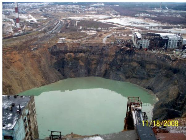
*Fig. 2. A salt collapse structure above the BKRU-1 mine.*
