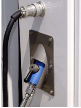
Figure 2. Hydrogen fuel dispenser at a filling station [8].
