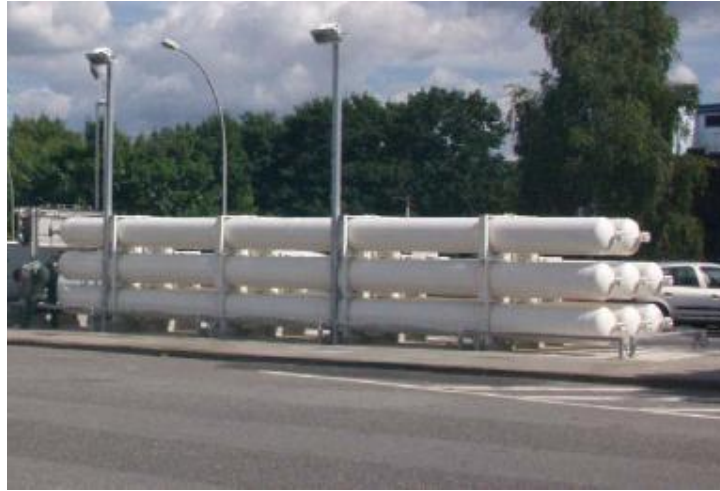
Figure 4. Stationary gaseous hydrogen storage [12].
