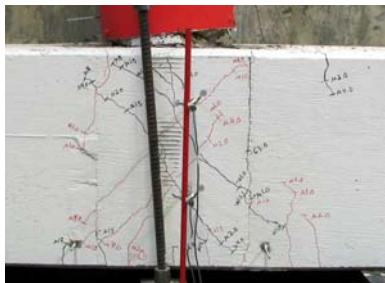
(b) Joint Damage
