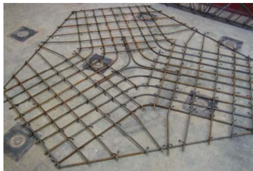
Figure 4.1. One Layer of Reinforcement for Footing and Slab
