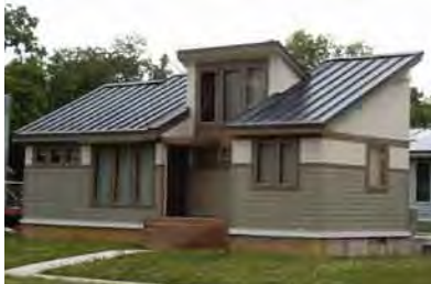
Solar Homes under construction
