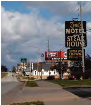
Existing Martin Springs Drive
