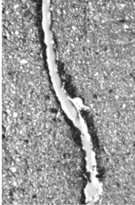
Figure 7-1 Crack Repaired by Routing and Sealing (ACI 345.1R 2006)
