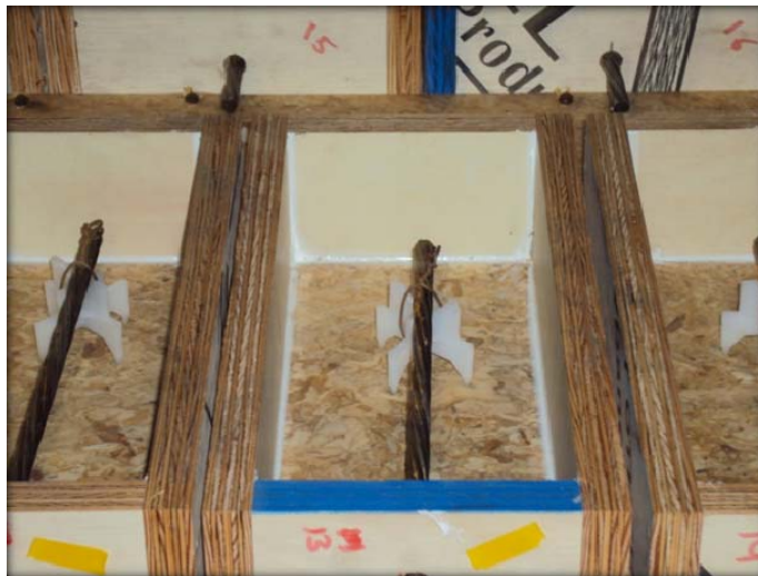
Figure C- 2 Non-Prestressed Corrosion Specimen - Formwork and Reinforcement
