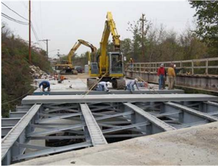
Figure 2-8 Fiber Reinforced Polymer (FRP) Deck Panel (Ralls 2005)
