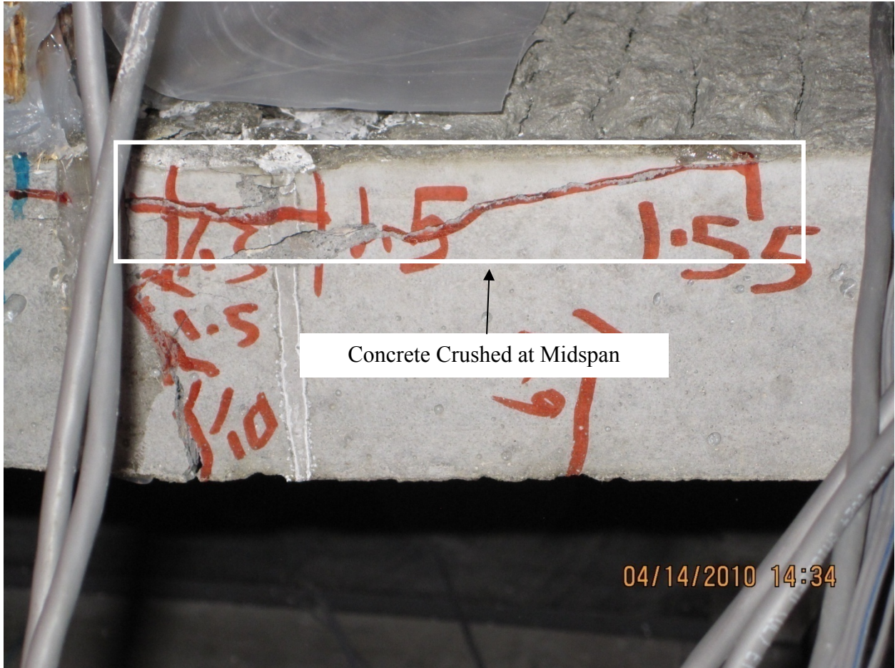
Figure C- 40 Flexural Failure at Midspan by Concrete Crushing of Panel CFRPT-NC-SL
