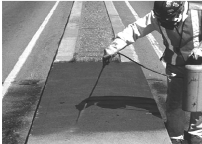
Figure 7-3 Application of Penetrating Concrete Sealer (ACI 345.1R 2006)
