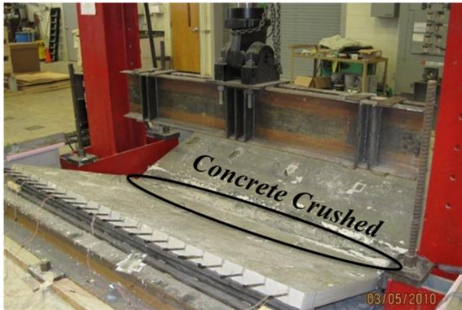
Figure 5-4 Typical Flexural Failure at Midspan by Concrete Crushing of Simply Supported Panels (Panel ST-NC-SL shown)
