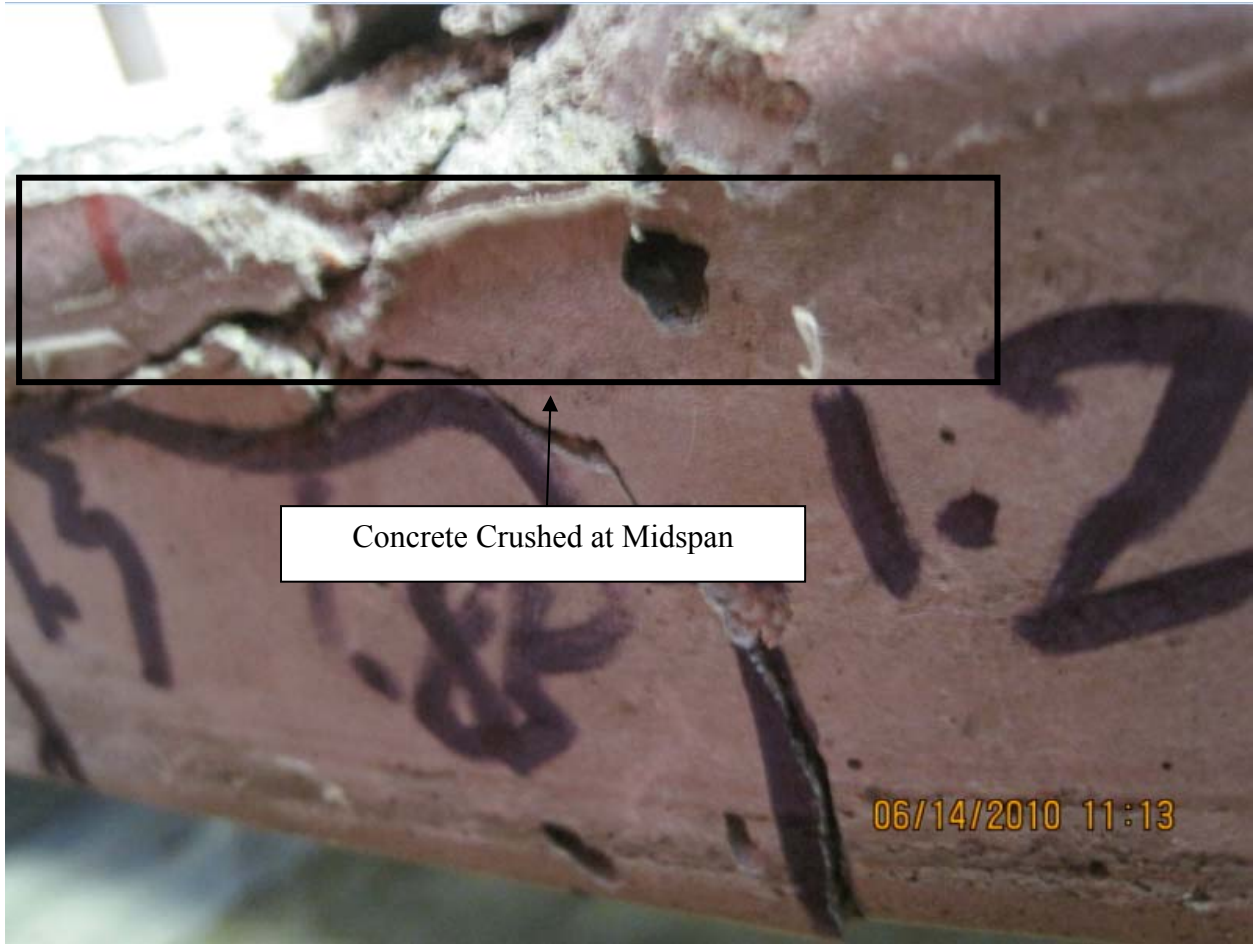
Figure C- 56 Flexural Failure at Midspan by Concrete Crushing of Panel ST-NC-FL
