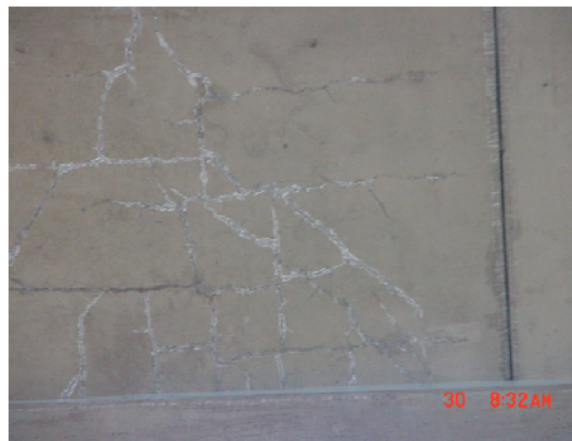
Figure 3-5 Cracking Observed in Colorado’s Partial Depth Precast-prestressed Concrete Panels
