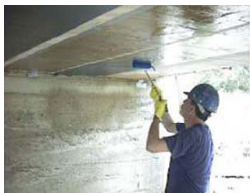
Figure 7-4 Application of the Adhesive to the Underside of the Deck (Mayo et al., 2000)
