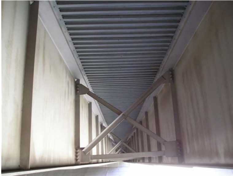
Figure 2-7 Bottom View of an SIPMF (Frost 2006)
