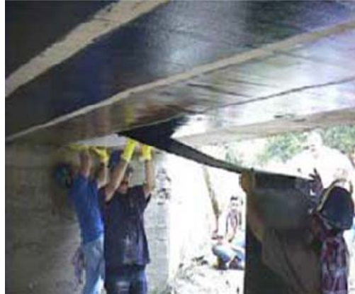
Figure 7-5 Installation of CFRP Sheets (Mayo et al., 2000)
