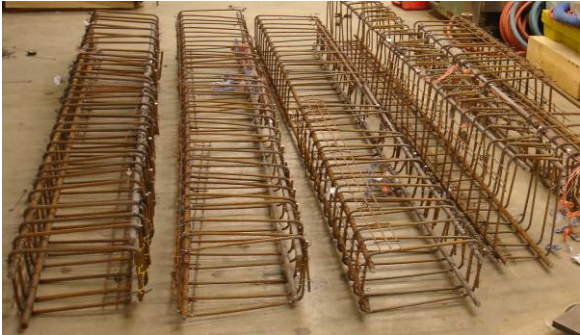
(a) Rebar cage of beams
