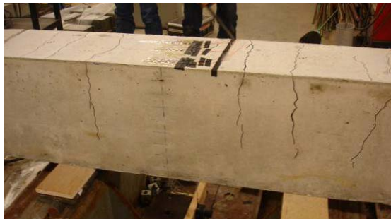
(b) Initial cracks
