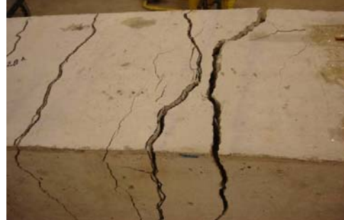
(c) Cracks at failure
