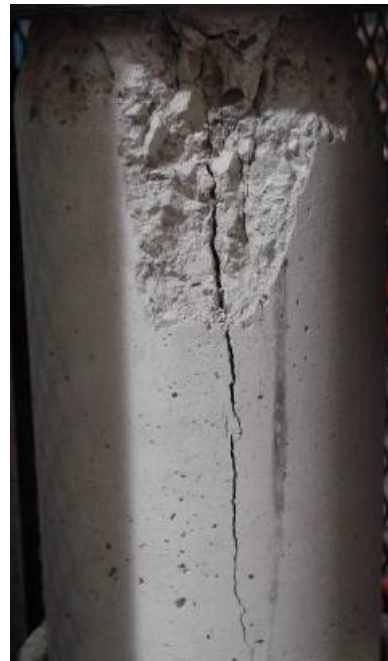
(b) Failure mode
