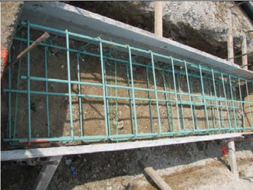
Sleeper slab reinforcement
