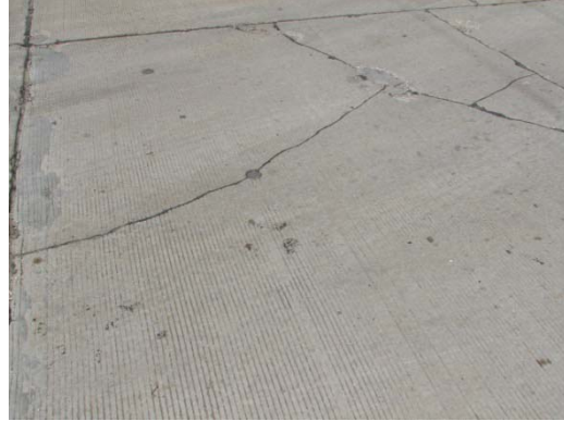
Surface cracking due to uneven settlement
