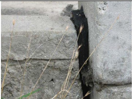
BAS movement from the abutment
