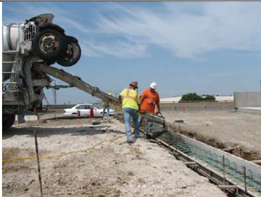
Pouring of Sleeper slab
