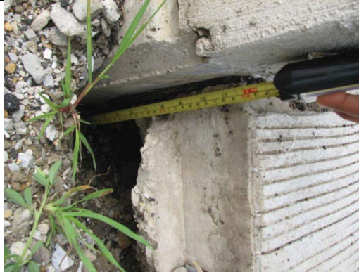
Erosion of soil underneath BAS
