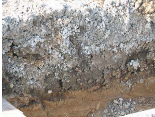
Approach slab base
