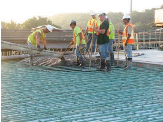
Pouring of Concrete in BAS
