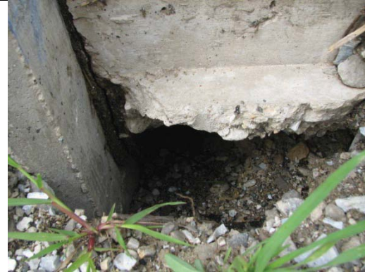
Erosion of soil underneath BAS
