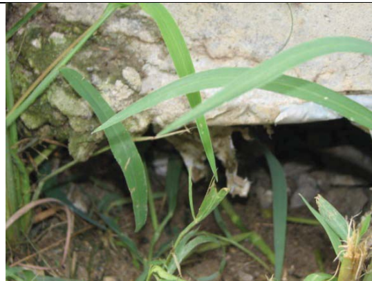
Erosion of soil underneath BAS
