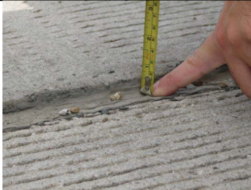
1/2" Bump at other end of the bridge
