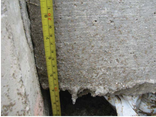
Soil erosion underneath BAS
