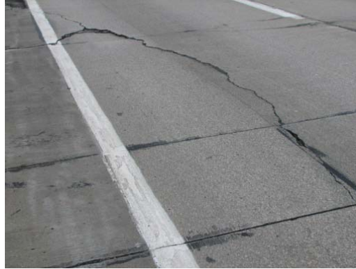
Surface cracking
