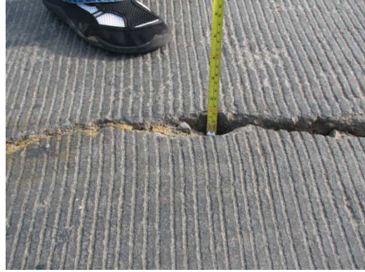
Surface cracking
