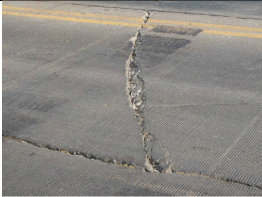
Surface cracking
