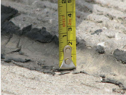
1" Bump at end of the bridge
