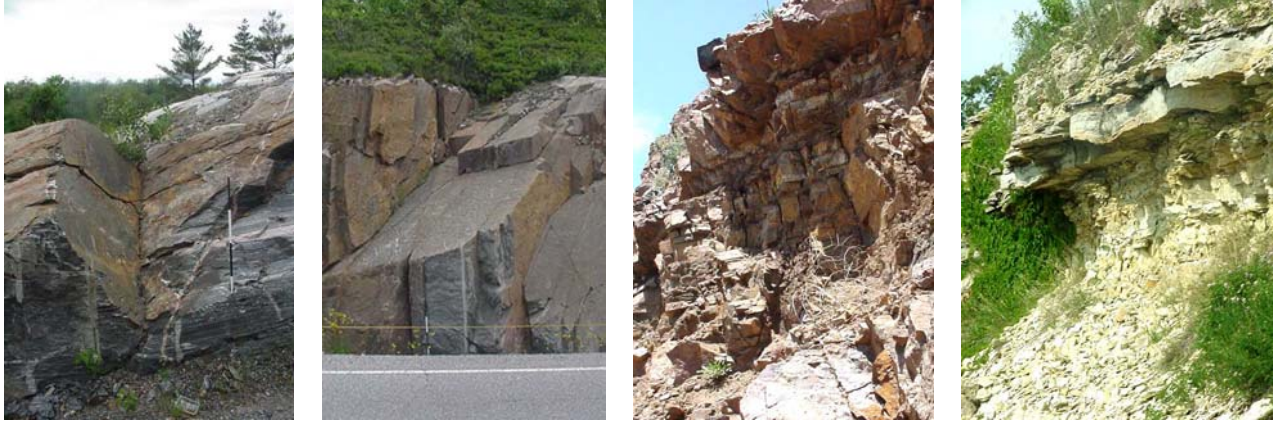
Figure 1: Example of wedge, planar, raveling, undercutting failures along road cuts.
