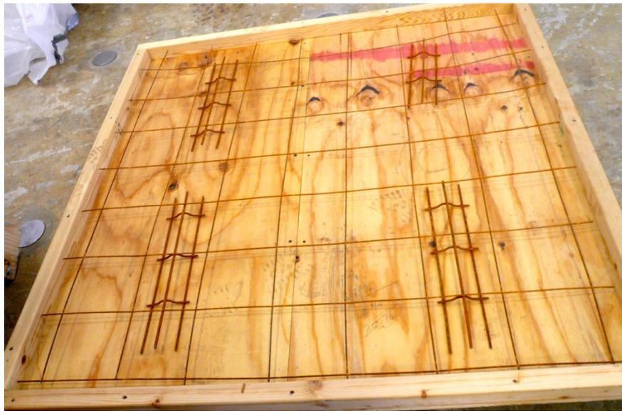
Figure 4.1: Impact Panel Formwork
