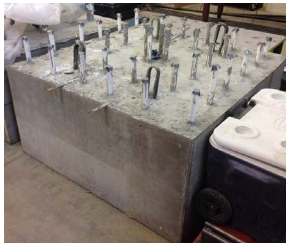
Fig. 3: Reinforced concrete footing of a self-centering bridge column that will be tested on the new shaking table.
