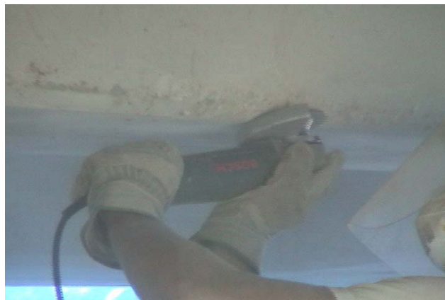
Figure 6. Rounding of corners on girder
