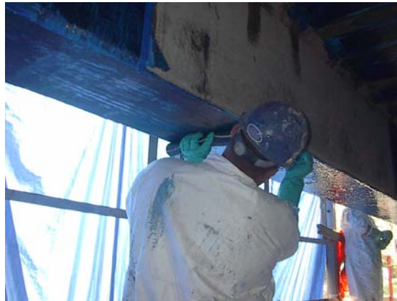
Figure 10. Manual lay-up CFRP sheet installation.
