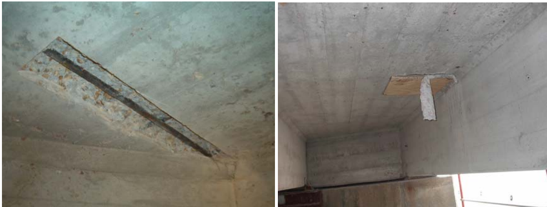
Figure 4. Repair of deteriorated areas on deck.
