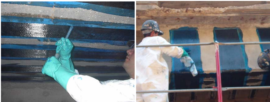
Figure 11. Squeezing of air bubbles and saturation over laminates
