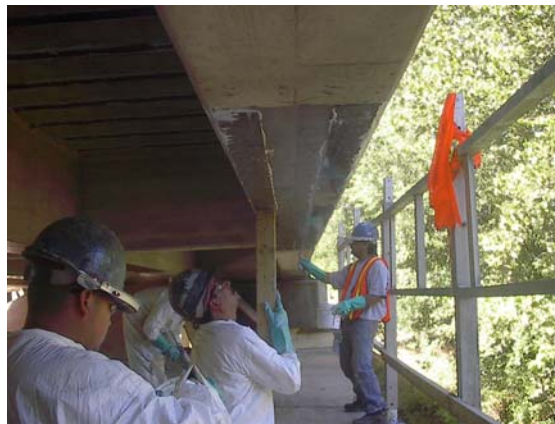
Figure 14. Installation of Pre-cured laminates
