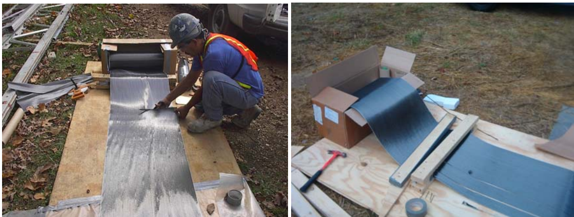
Figure 9. Cutting process of CFRP sheet
