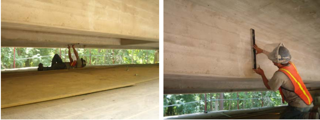
Figure 5. Levelled of surface
