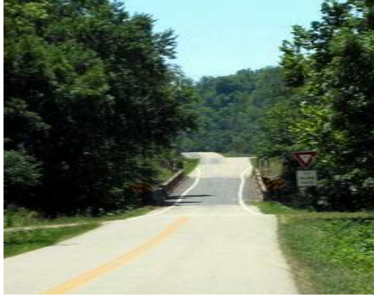
Figure 1. Approach to the bridge
