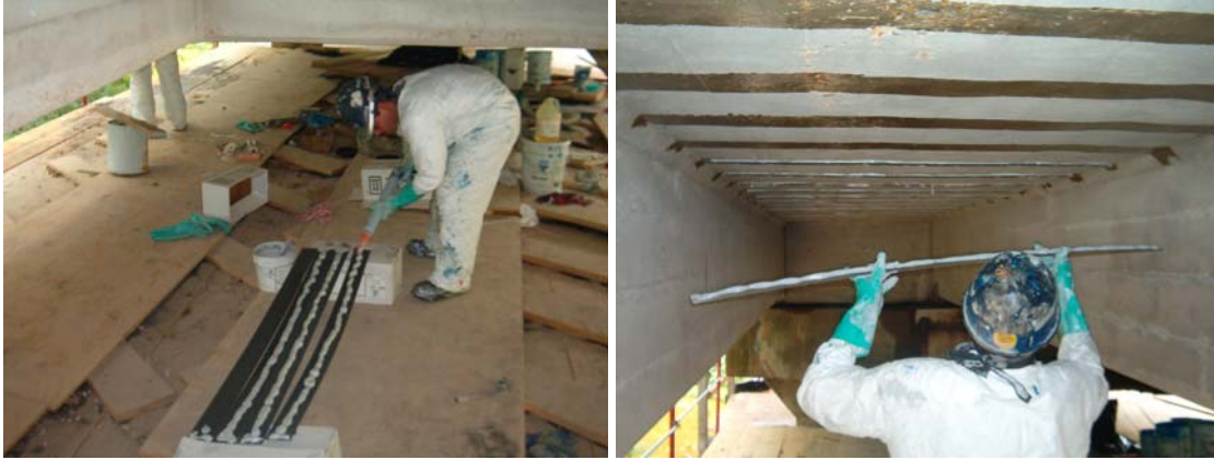
Figure 13. Installation of Pre-cured laminates
