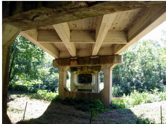
Figure 2. Longitudinal and transversal beams
