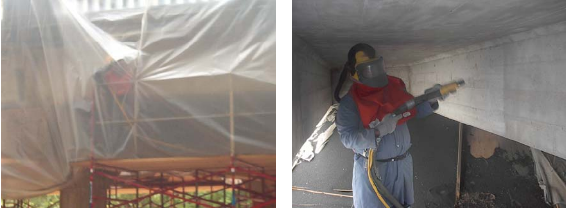
Figure 7. Preparation of appropriate roughness by sandblasting
