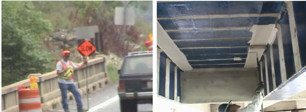
Figure 12. Traffic control and topcoat protection
