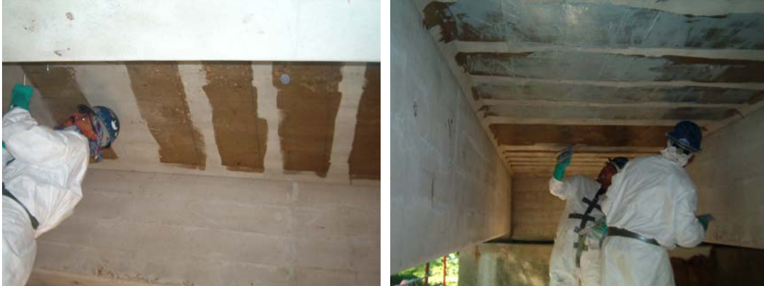
Figure 8. Filling of voids and defects by primer and putty collocation
