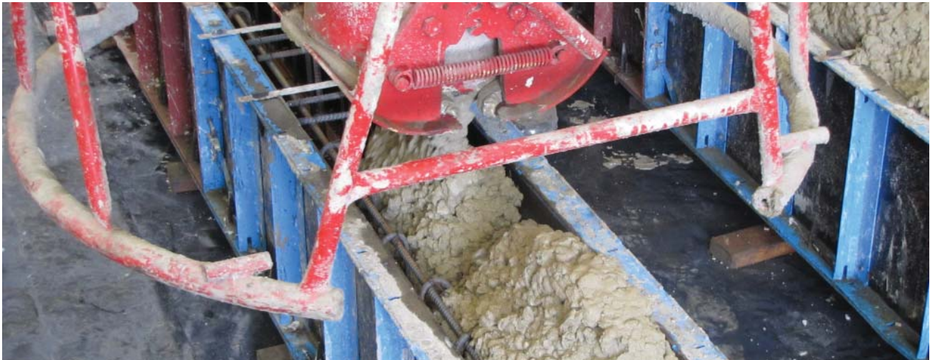
Figure 1. Construction of high-volume fly ash concrete full-scale test beams
