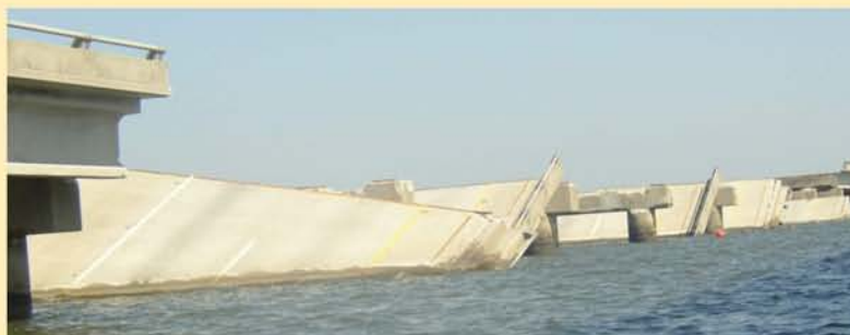
Fig. 2 Major damage to approach structures: drop-off spans and excessive lateral displacement
