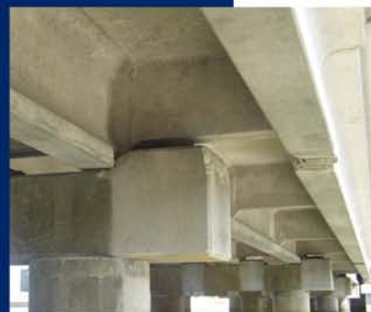
Fig. 1 Typical cross section and diaphragms underneath the bridge decks
