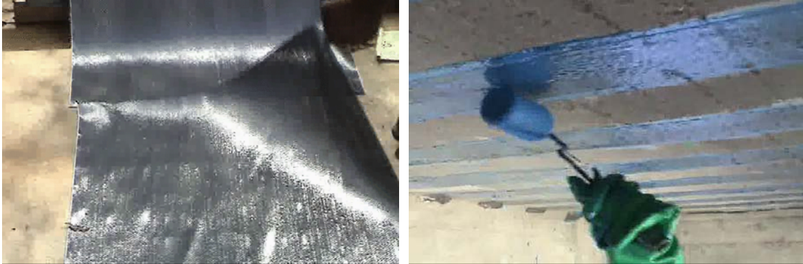
Figure 5. Cutting process and saturant application
