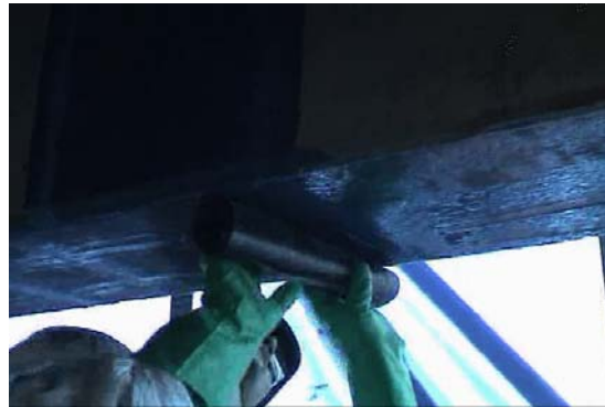
Figure 6. Manual lay-up CFRP sheet installation.
