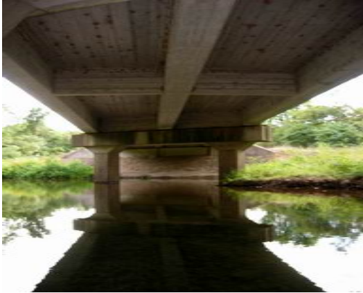
Figure 3. Condition of deck
