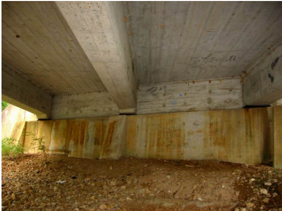
Figure 2. Condition of abutment
