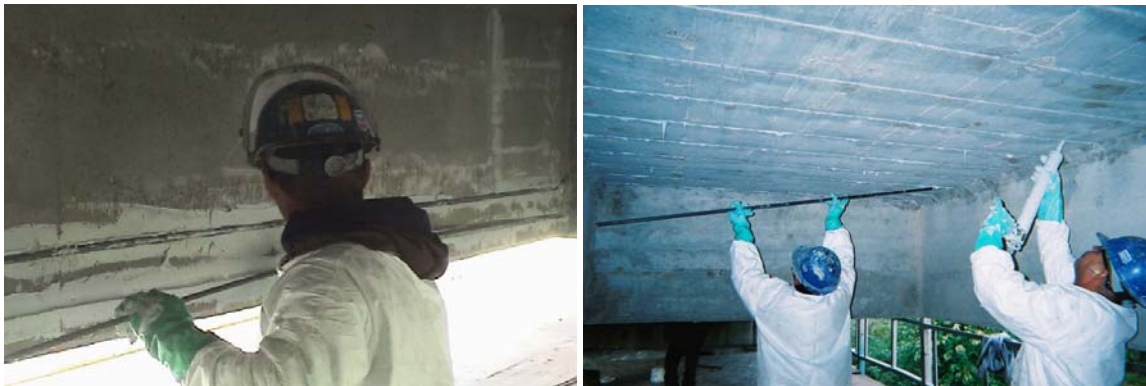
Figure 10. Bar installation on girder and slab
