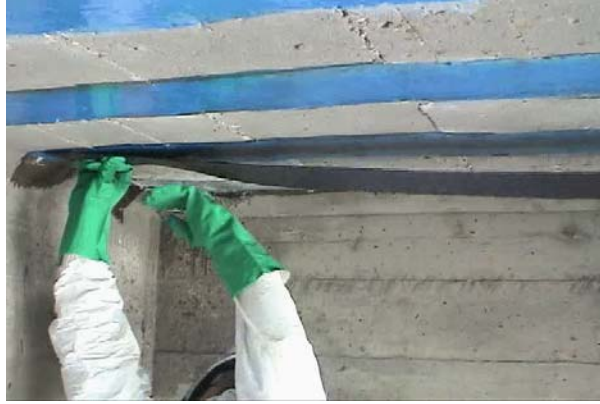
Figure 7. Manual lay-up CFRP sheet installation.
