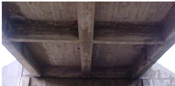
Figure 3. Condition of deck
