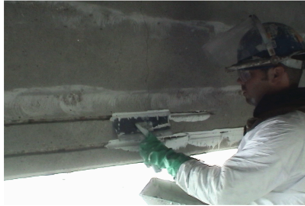
Figure 9. Epoxy adhesive in slot cut in the concrete surface
