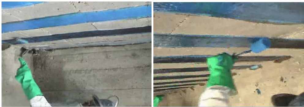
Figure 8. Squeezing of air bubbles and saturation over laminates
