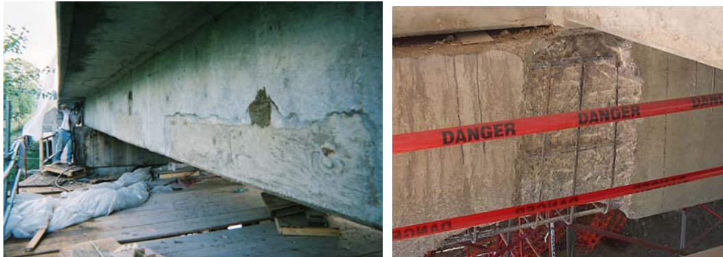
Figure 4. Repair of deteriorated areas on girder and bent
