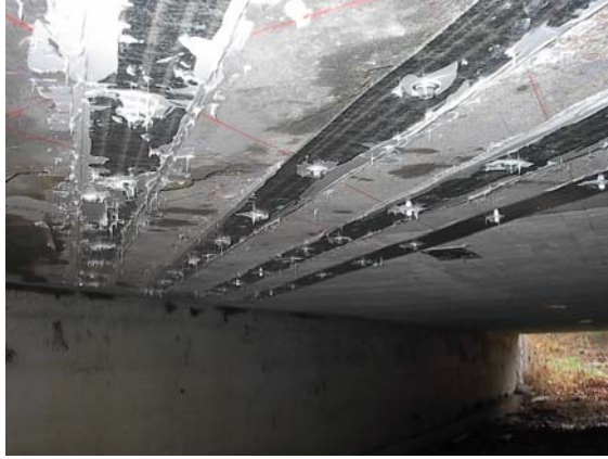
Figure 8. Installed mechanically fastened laminates.
