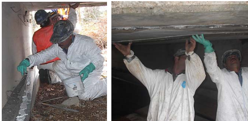
Figure 5. Installation of mechanically fastened laminates
