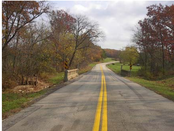
Figure 1. Approach to the bridge
