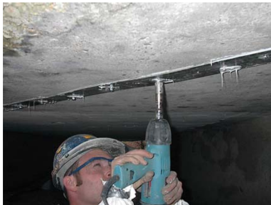
Figure 7. Installation of fasteners
