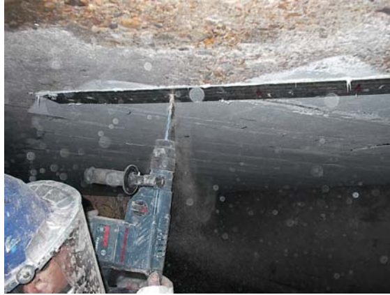
Figure 6. Drilling of laminates and concrete surface.
