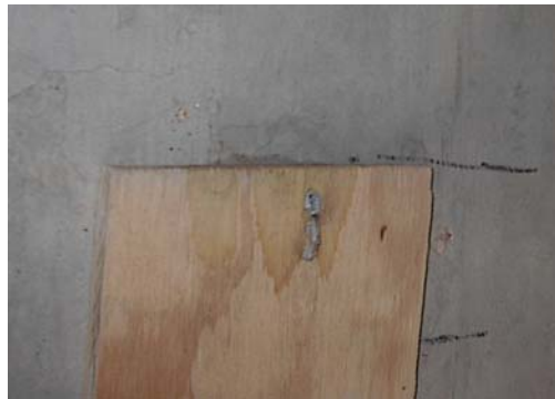
Figure 4. Repair of deteriorated areas on deck
