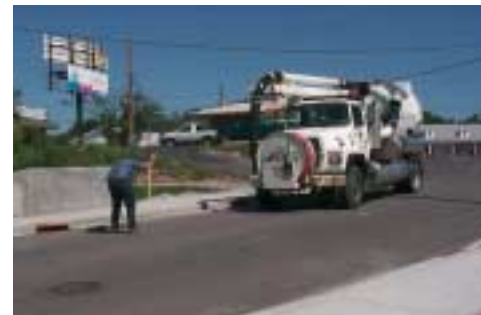
Figure 13. In-situ load test
