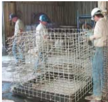
Figure 3. GFRP cage
