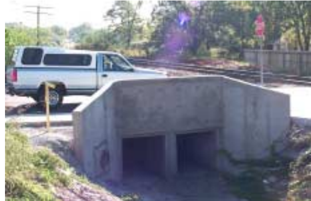
Figure 11. New Walker Avenue Bridge
