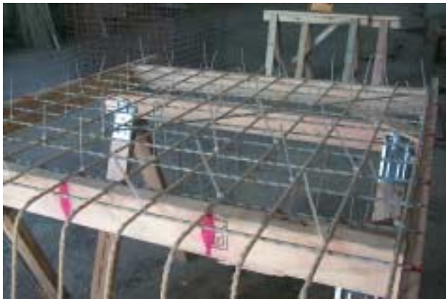
Figure 2. Rig for GFRP cage assembly
