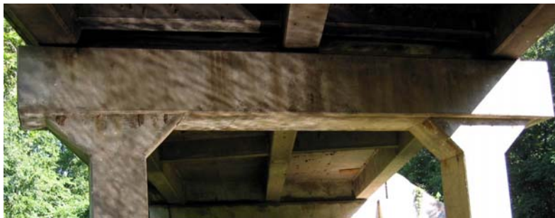
Figure 2 – Superstructure of the Bridge
