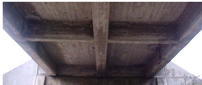
Figure 2 – Superstructure of the Bridge
