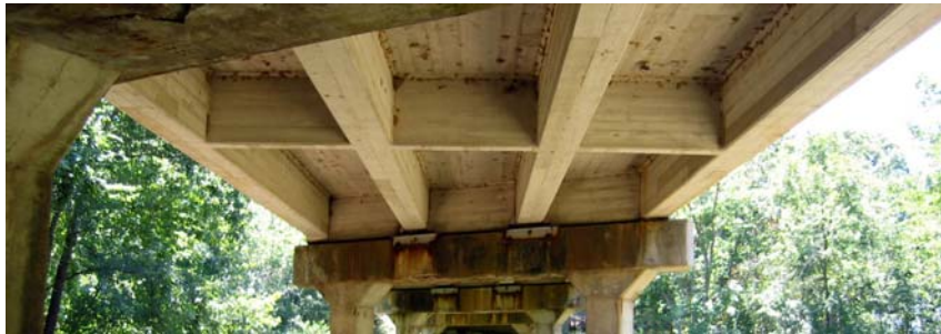
Figure 2 – Superstructure of the Bridge
