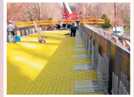
Construction of Greene County Bridge
