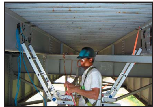
Strain gage installation
